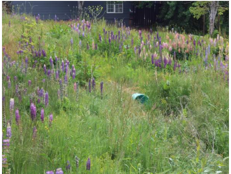
Part of the solution - this detention basin along Doaks Ferry Road NW is designed to treat water quality as well as retain storm water
